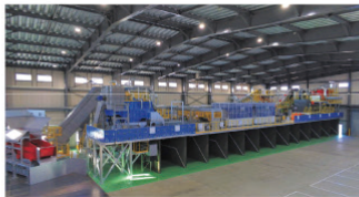
Construction-type waste disposal plant
