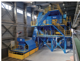
Building B, JR East Resource Recycling Center
